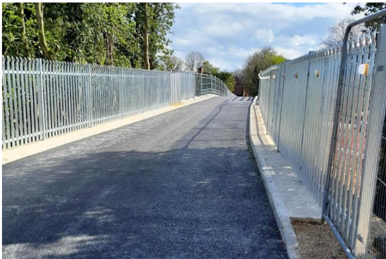
Network Rail completes footbridge over Midland Main Line for electrification project | New Civil Engineer
